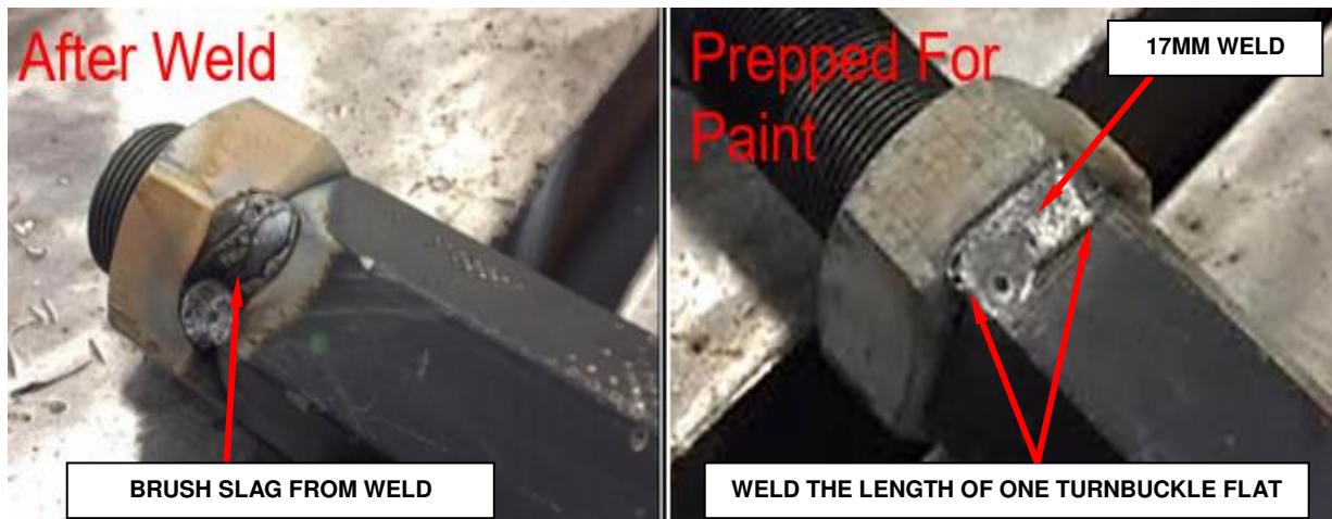
Figure 10 – Prepare areas for Paint
