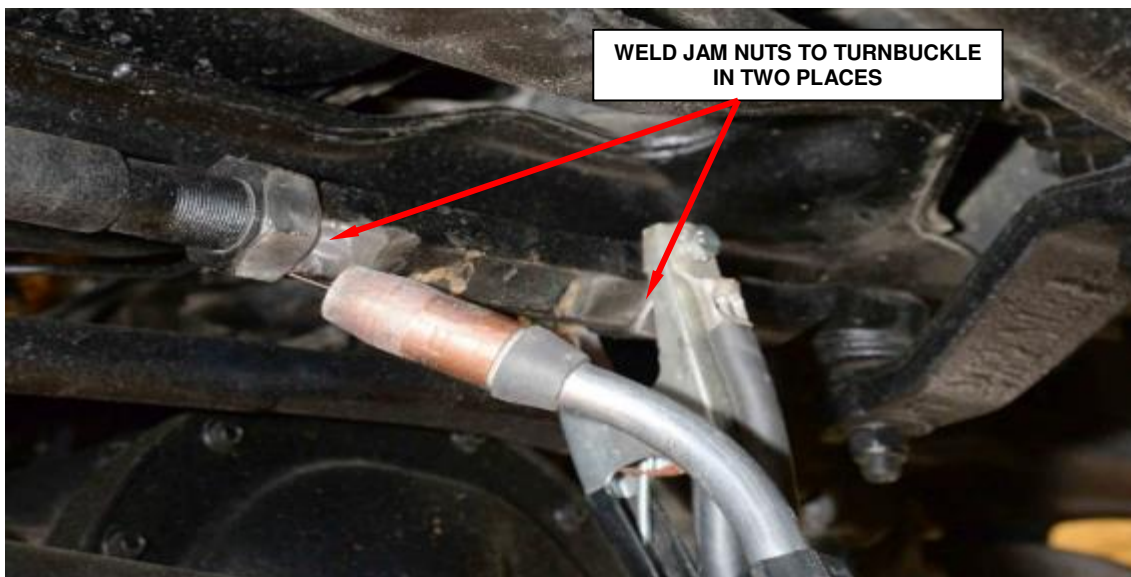
Figure 9 – Weld Both Jam Nuts to the Turnbuckle
